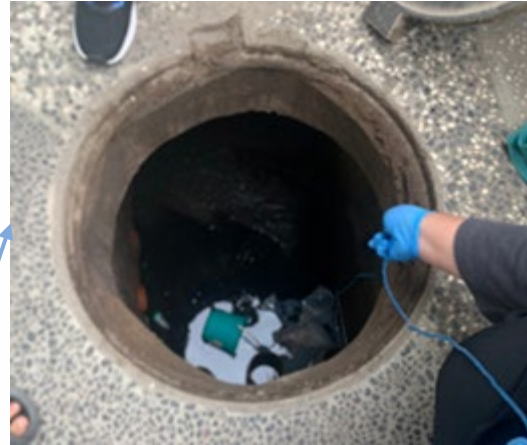
Take wastewater samples using a bucket
